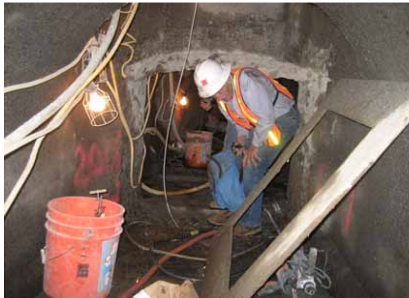
Figure 14. Enlarging concrete breast-wall for gate thimble.
