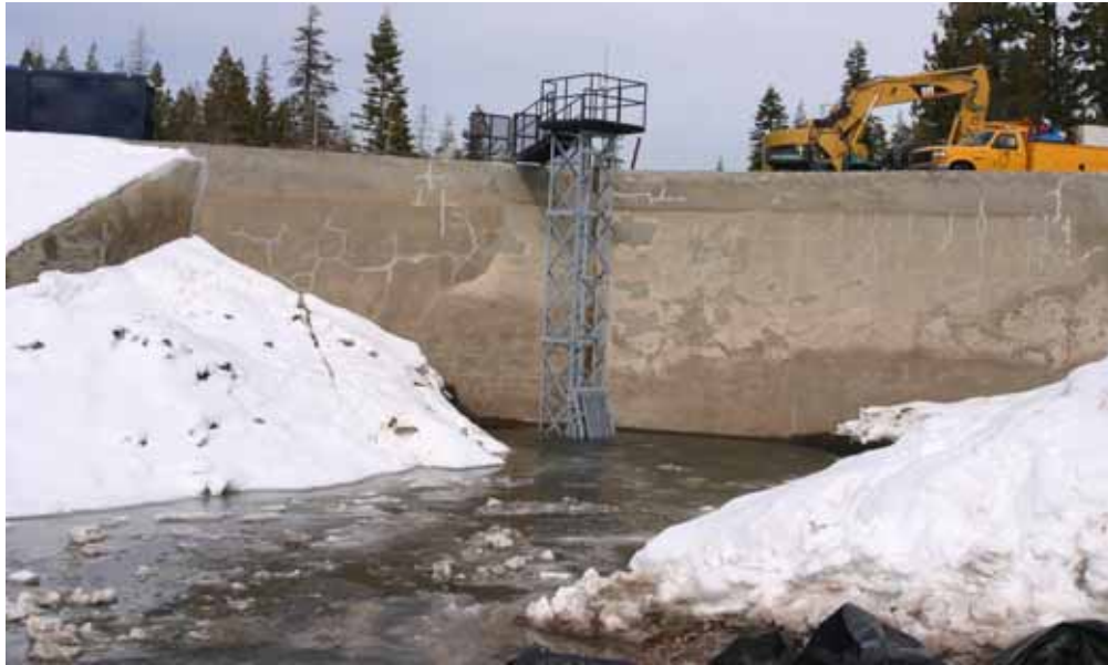
Figure 16. Completed Silver Lake emergency tower and gate replacement
