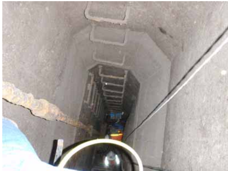
Figure 13. Working within 68 ft. deep, tapering, cramped gate wet well shaft.
