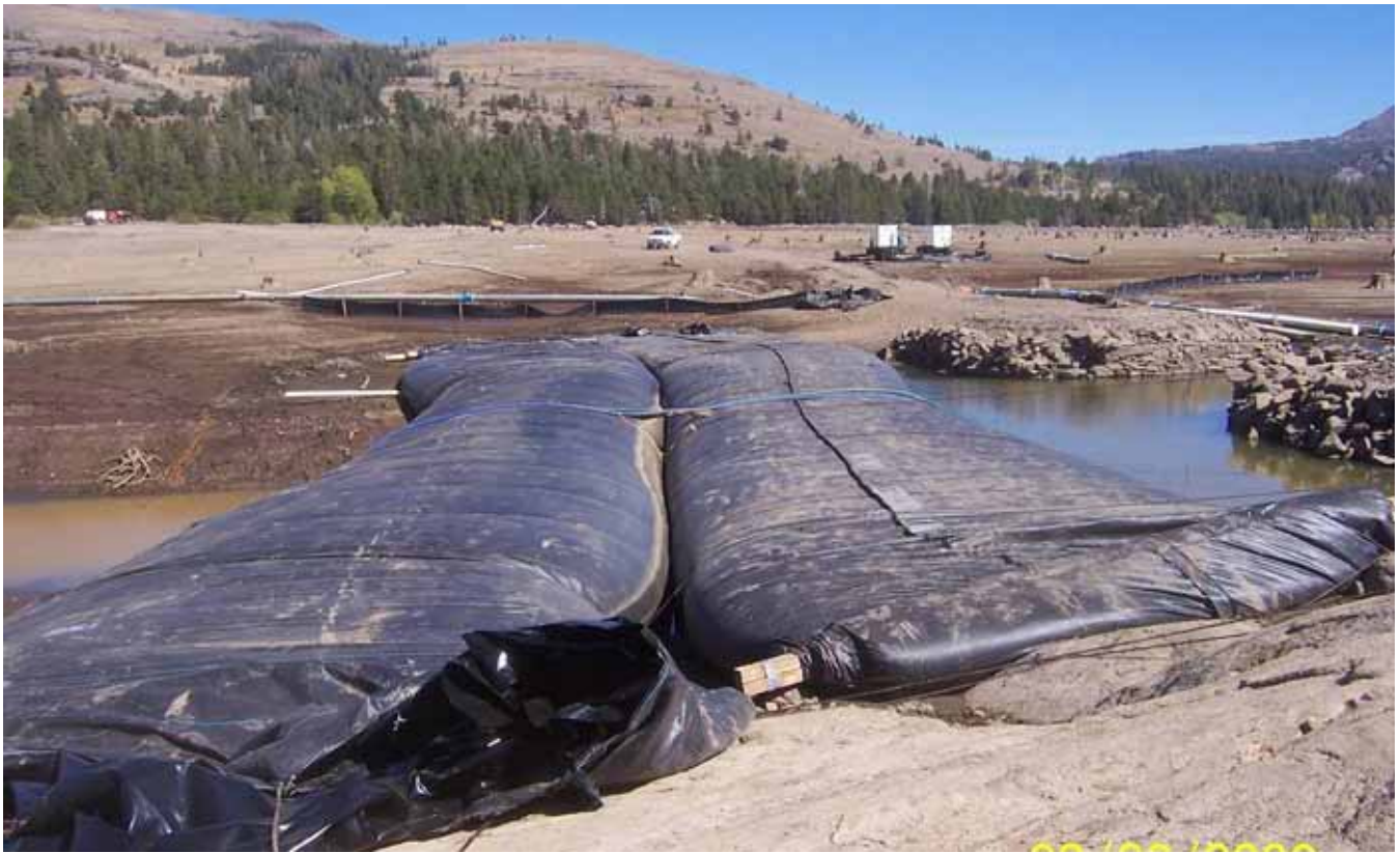
Figure 9. Bladder dams for the 2008 emergency repair of Caples Dam outlet
