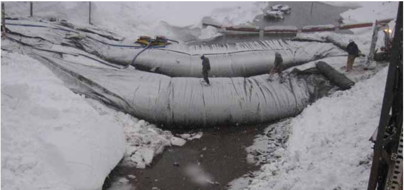
Figure 10. Bladder dams for the 2009 emergency repair of Silver Lake Dam
