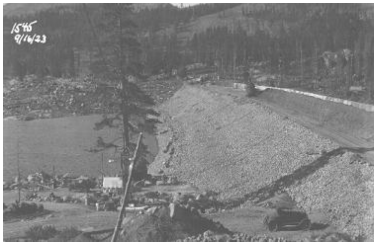
Figure 2. Caples Lake Main Dam during raising, 1923.
