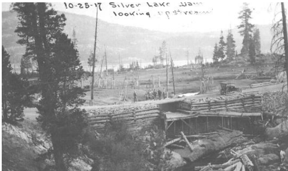
Figure 3. Silver Lake Timber Crib Dam as constructed in 1917.
