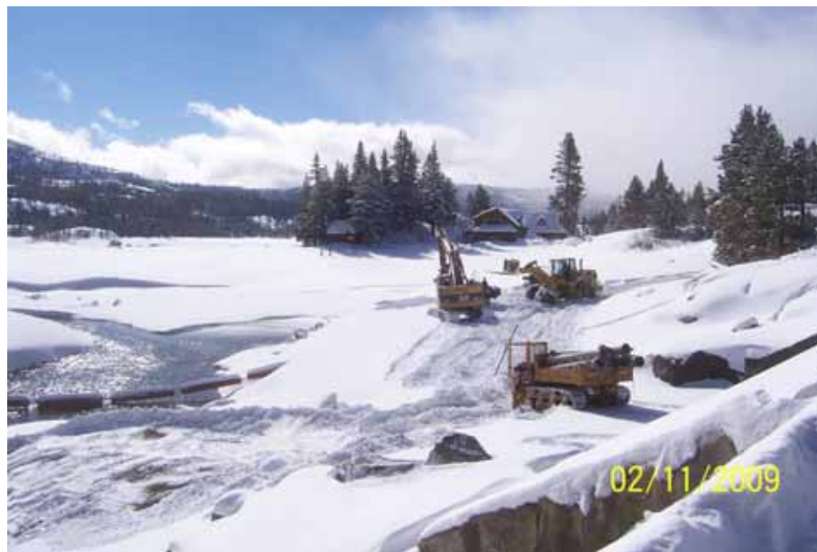
Figure 15. Construction site during 2009 emergency repair of Silver during good weather
